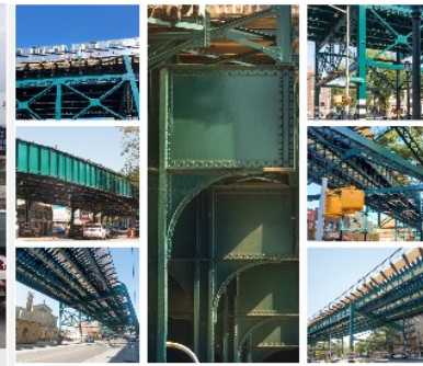
Painting of Elevated Structures on the #7 Line
