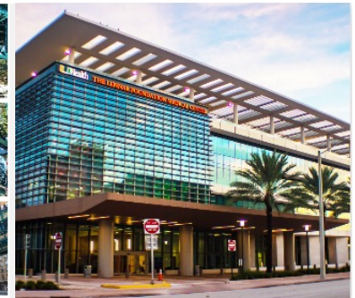
UHealth Lennar Foundation Medical Center
