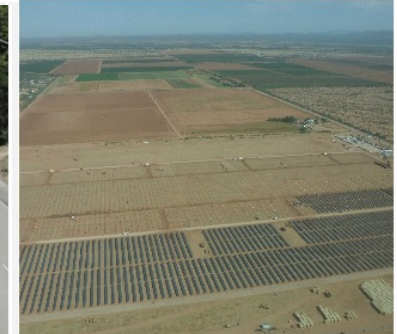
Tucson Solar Power Plant
