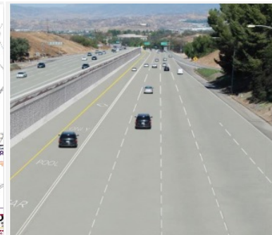
I-5 North Freeway Enhancements
